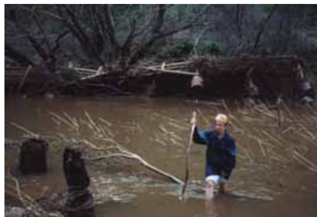
Barb Jeffrey and the remains of the bridge Photo: Graham Jeffrey, 2 Sept, 1992
